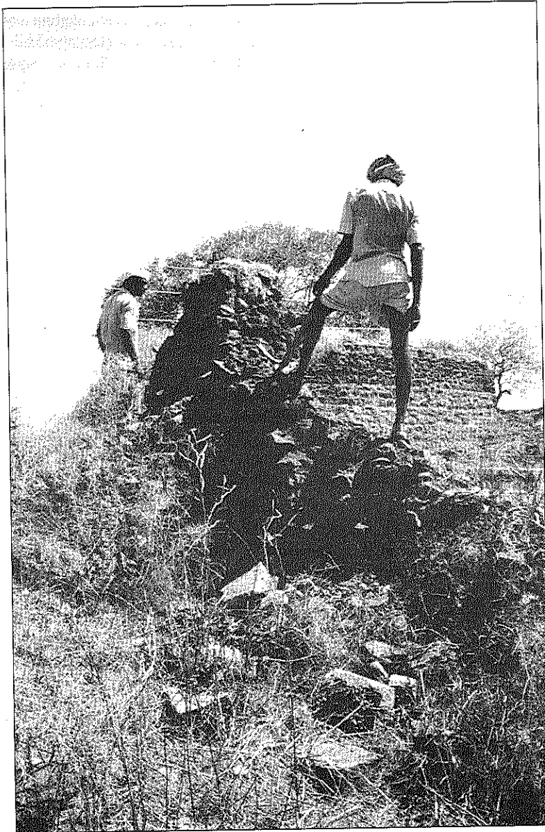
Figure 4.4: Reconstruction Work at Banegaon Village
